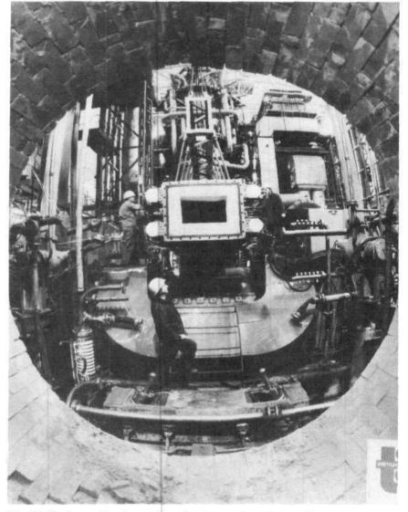
The MHD channel in the gas-burning Soviet U-25, the world's first pilot MHD plant.
